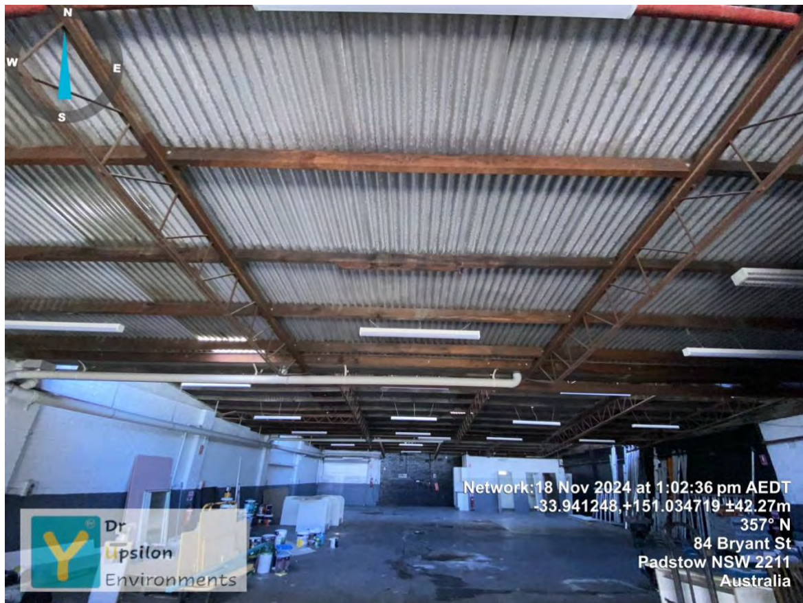
Figure 1 The site at 86 Bryant Street, Padstow, NSW
